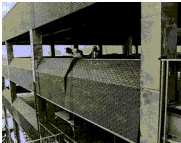
Positioning Prefabricated Panel
