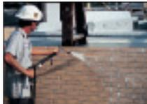
Panel is cleaned to remove concrete leakage.
