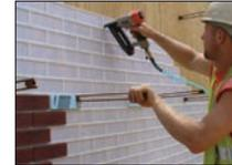
Rim snaps tab together and are stapled on a vertical surface to create a template to hold brick.
