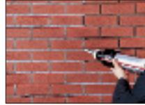
Mortar is installed into the brick joints with a grout bag or with mortar dispensing gun.
