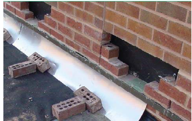
Photo 3 Flashing Installed in Alternating Sections
