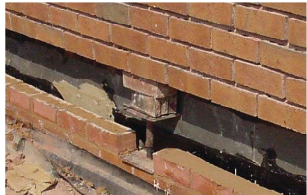
Photo 4 Flashing Installation Using Temporary Support
