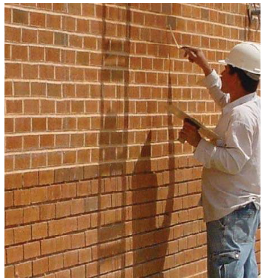
Photo 2 Repointing Mortar Joints
